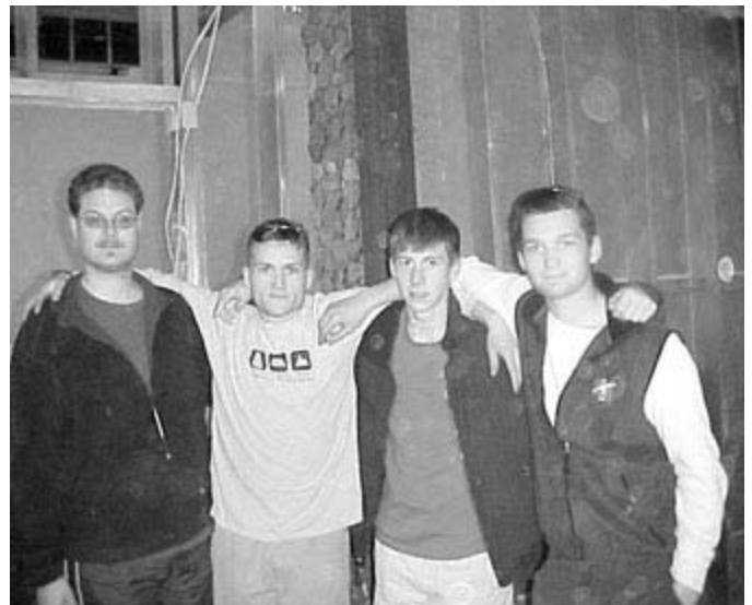
Winter Wonders! Staff Adviser Matt Randall, Paul Beaupre, Tom Parenteau, and Lodge Chief Paul Froman shine in front of the renovations taking place at the Rotary Training Center.
